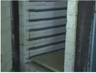
The new kiln
